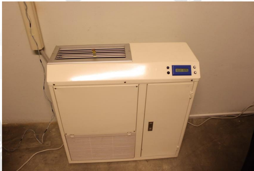
Figure 1. A precise climate controller with the dimension of 0.3 x 1.0 x 1.2 m (W x L x H) which is similar to a 10,000 BTU air condition.
